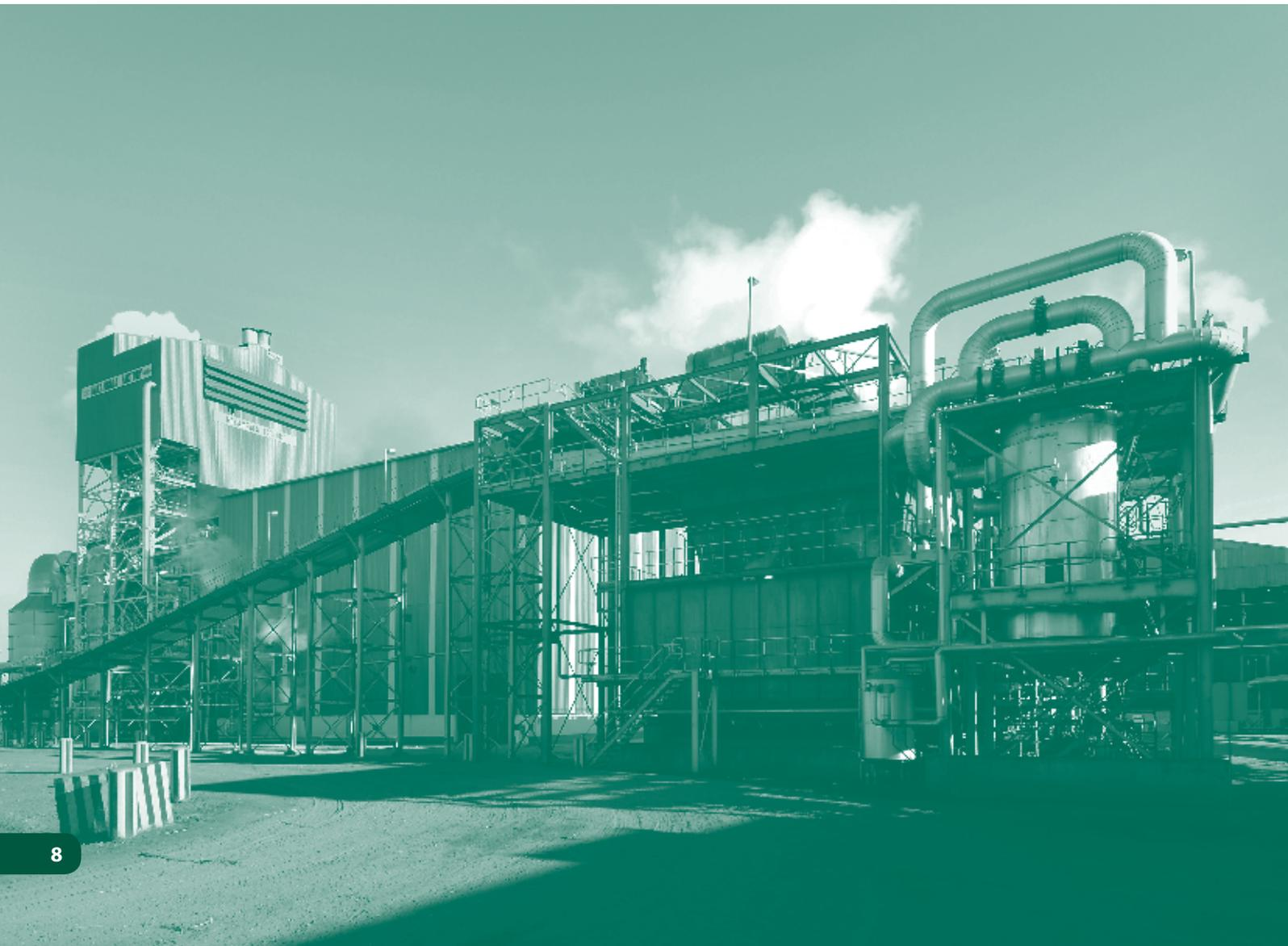
bagasse. Emission levels of sulphur dioxide and nitrogen oxides are low compared to conventional fossil fuels due to the characteristically low levels of sulphur and nitrogen contained in bagasse. The new boiler installed during the expansion project is fitted with a wet scrubber, which serves to remove almost all the particulate matter and gas from emissions into the atmosphere.
